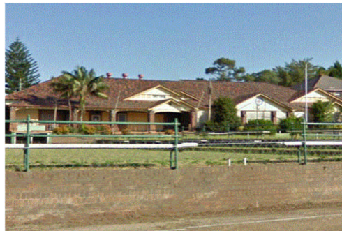
View of existing building Samples A1 to A3 Looking northwest
