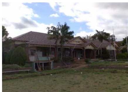
St George Bowling Club House Looking north east
