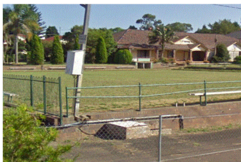
View of existing building Samples A4 to A6 Looking northwest
